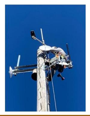
The equipment rack inside the shelter is used to house the router, network servers and the switches. The tasks of the day were to add another parabolic dish to the tower for 900 Mhz and to align it the antenna at the Elliot hospital in Manchester. Another 5 Ghz dish was also fine tuned in azimuth and elevation toward the Westford node of the network.
