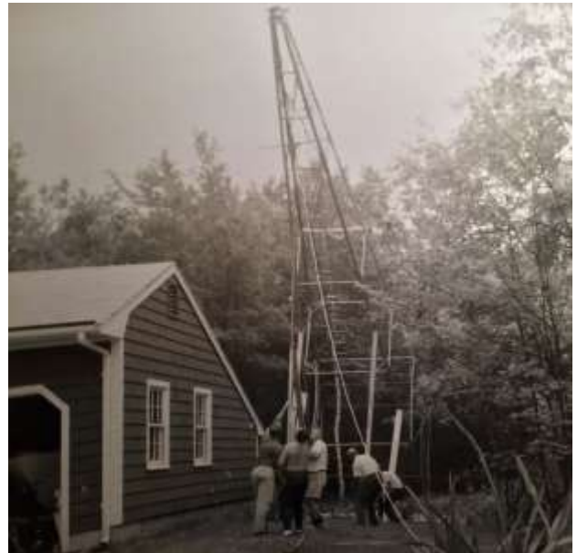
Erecting the Tower
