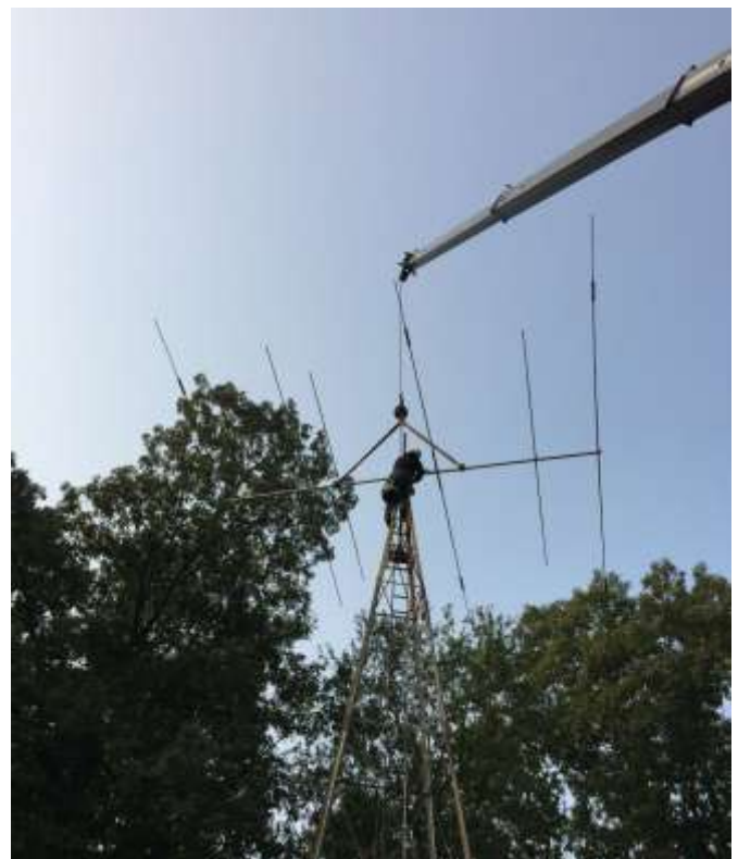
Removing the Beam
