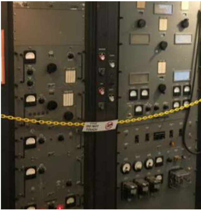
Figure 9. RCA SSB-T3 Type-H 2-30 MHz 20 kW Transmitter of the Type Used Circa 1978-1998
