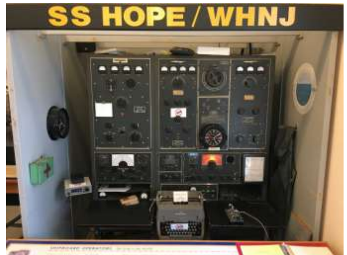
Figure 11. An Example of a Shipboard Radio Station
