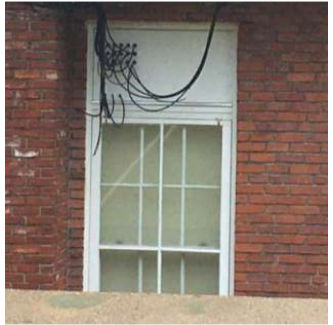
Figure 15. WAIWCC Antenna Cables to Antenna Trail at Chatham Marconi Center
