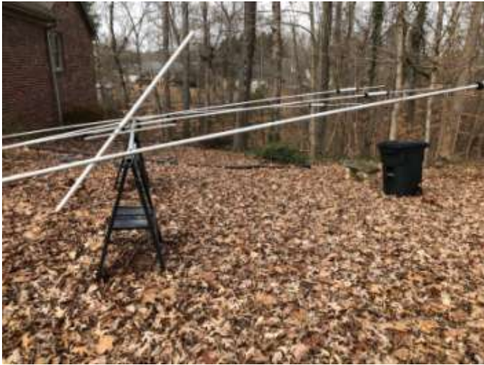
Figure 1: Elements Roughed-in But Definitely Not in Any Sort of Alignment
